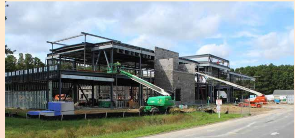
New construction on the campus of Eastern Shore Community College.
